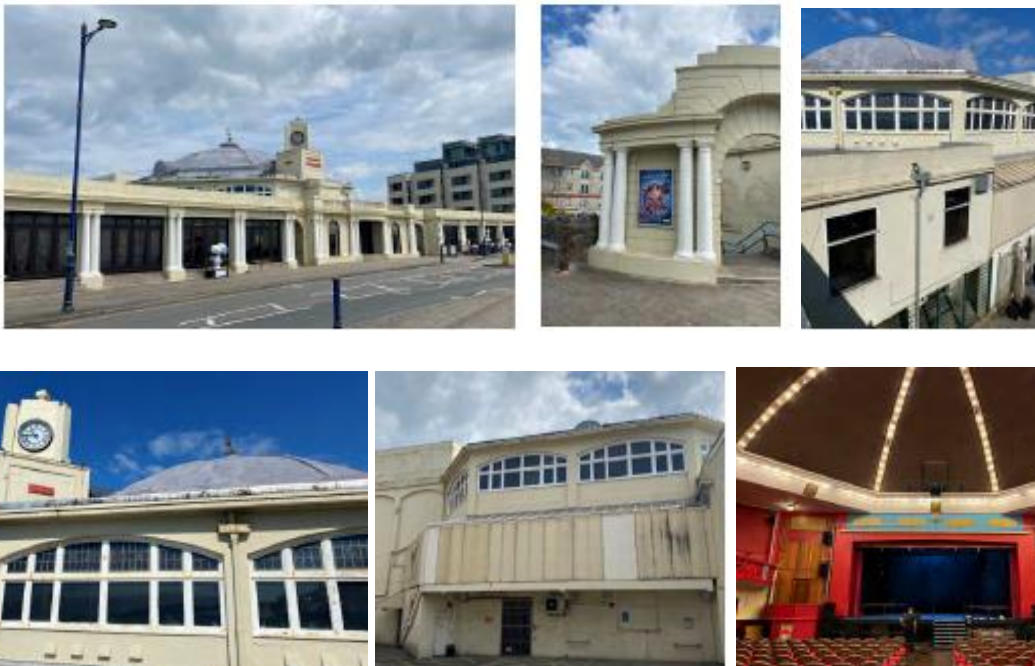
Figure 8 – Photographs of the application building
