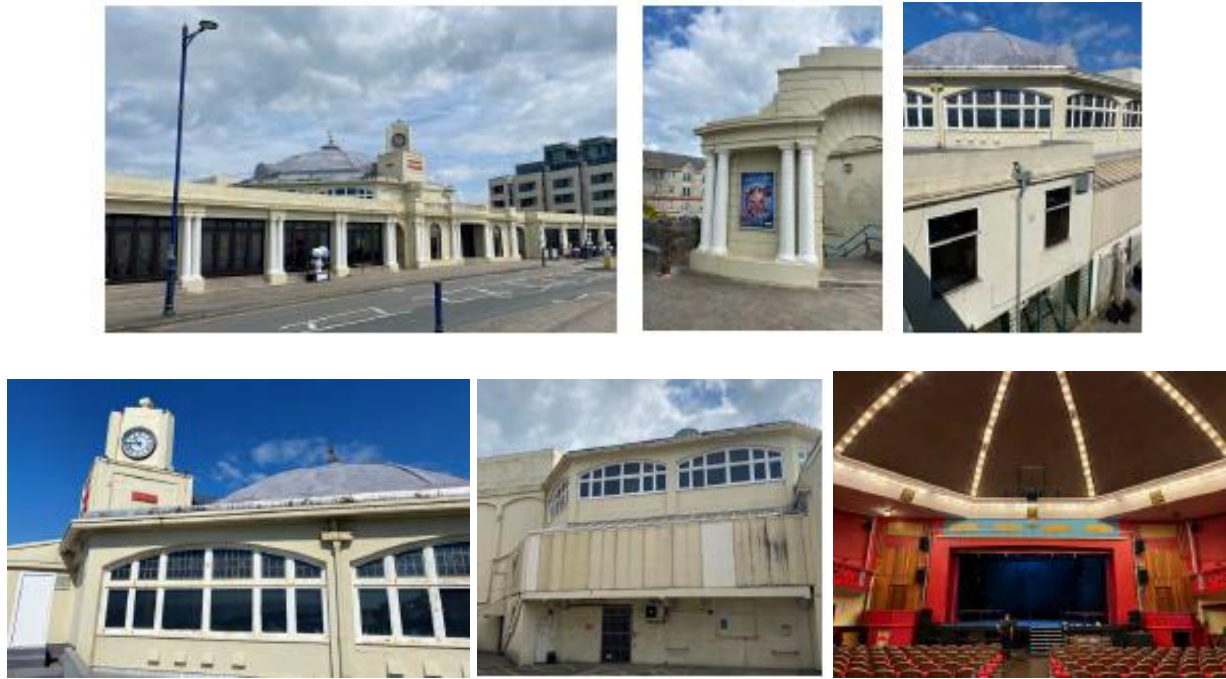
Figure 8 – Photographs of the application Building
